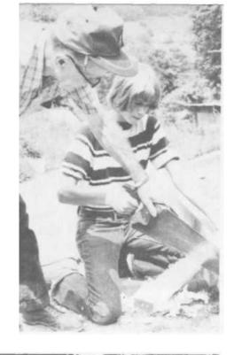
PLATES 176-177 Tedra nails a metal strip to the front of each runner, then he fits the front end of the half sole into it and bends it over to fit the runner's curve.
