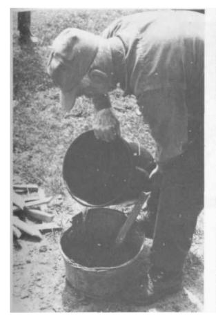
PLATE 256 The water was poured onto the clay, then stirred to make a good stiff mixture.
