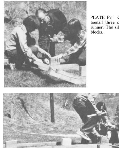
PLATE 165 Cheryl and Dwayne Skenes toenail three chestnut blocks onto each runner. The sills will fit on top of these blocks.
