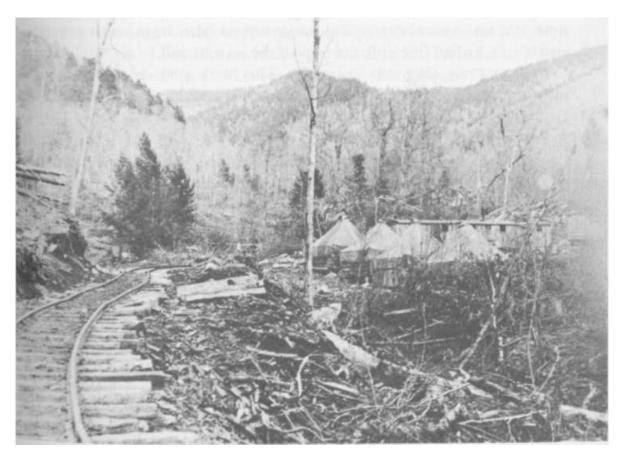
PLATEE 287 Another logging ramp, this one at the head end of a narrow-gauge rail-O line. The dwellings are log sides with canvas roofs. The long, narrow wooden building behind the dwellings is probably the cook shack. An operation like this one night have seventy-live to a hundred men living there at one time. (Photo courtesy of ChampionPaper)
