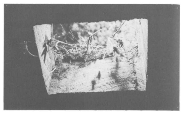
PLATE 323 A 10"X 12" vent for condensation, from the inside looking out.
