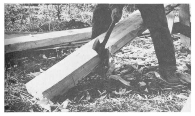
PLATE 409 From the center of the log, he measures off the width he wants the beam to be, flips two chalk lines as guides, raises the log onto sawhorses, and slices off the sides with an axe. He first scores the sides, then goes back and hews to the line.
