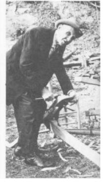
PLATE 155 Here Tom attaches the metal plow point to the foot with a bolt.
