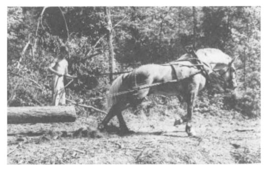
PLATE 266 When the logs are hooked together, Millard's horse, Charley, is backed up to the lead log and chained to it via the singletree at the end of his harness, and a "J-grab" or "header grab" that connerts the singletree to the lead log. At a signal from Jack, Millard's son, Charley lunges forward to get the train of logs moving.
