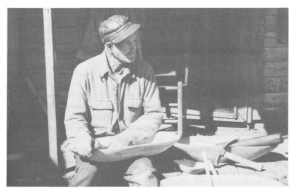
PLATE 109 Finally, using the hammer and chisel, Alex hews out the outside surfaces, and then doits the final shaping and smoothing with a wood rasp and sandpaper.
