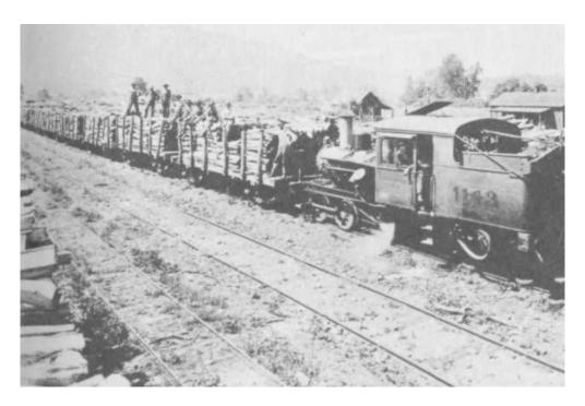
PLATE 273 This photograph shows acid wood being moved into the plant's yard by narrow-gauge railroad. The engine, called a "little Shay," pushes twenty-five to thirty "dinky cars" at a time, each loaded with six to eight cords of wood. (Photo courtesy of Champion Paper.)
