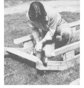
PLATE 168 A hole is drilled through each end of the crosspiece into the runners below, and pegs inserted. Here, Louise Freeman saws the yellow locust, pegs off flush.
