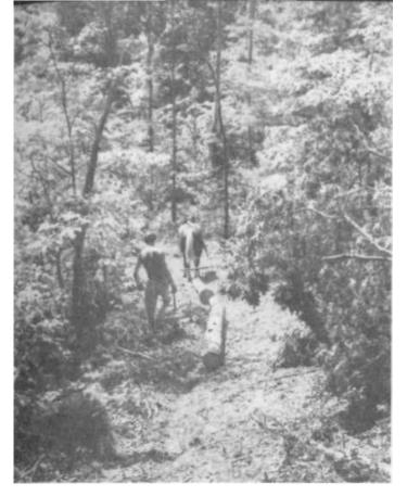
PLATE 267 The logs arc dragged down a skid trail to the truck. Dogwood posts are driven into the ground at intervals to back up small fender poles along the downhill edge of curves in the trail which keep the logs from rolling out. Such skid trails are still visible, more than thirty years later, throughout the mountains.
