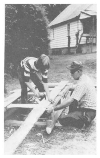
PLATE 182 After the other half sole is set the sled is righted and an oak floor is added. With the standards replaced, it's ready to use. Some farmers also make a long wood box with high sides that will fit down between the standards and rest on the floor. This is set on the sled when hauling small rocks, corn, and the like, and is removed when not needed.
