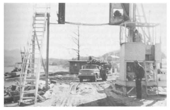
PLATE 280 A loaded truck approaches a saw that cuts the logs in half while they arc still on the truck.
