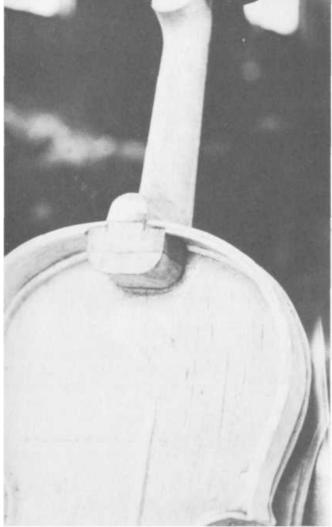
PLATE 117 The neck of the fiddle has been cut out of a block of maple 9"X21/4"X21/4". It is shaped with a pocketknife and sandpaper. The end may have any design you want. Pegs are tapered so they will tighten in their holes.
