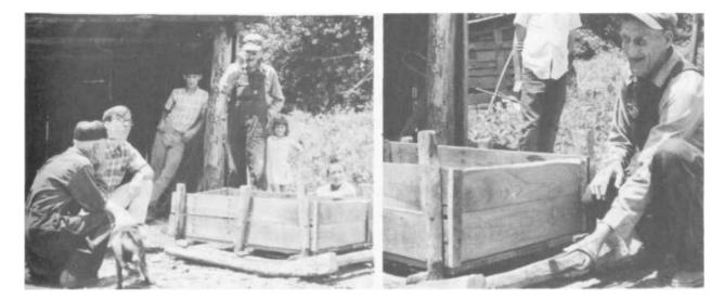
PLATES 193-194 (Variation #4) This sled was made by Harv Reid in Blairsville, Georgia. It has curved sourwood runners and a mortised crosspiece, but the box is nailed to the standards and rests on crosspieces that are nailed to the tops of the runners. In Plate 194, Harv shows where the clevis goes.
