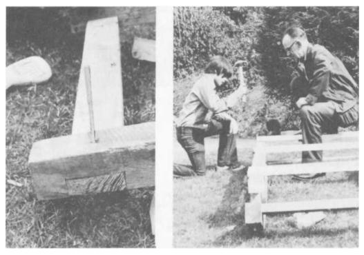
PLATE 170 When the wedge is in place, as shown here, again a saw is used to cut it off flush with the bottom of the runner.
