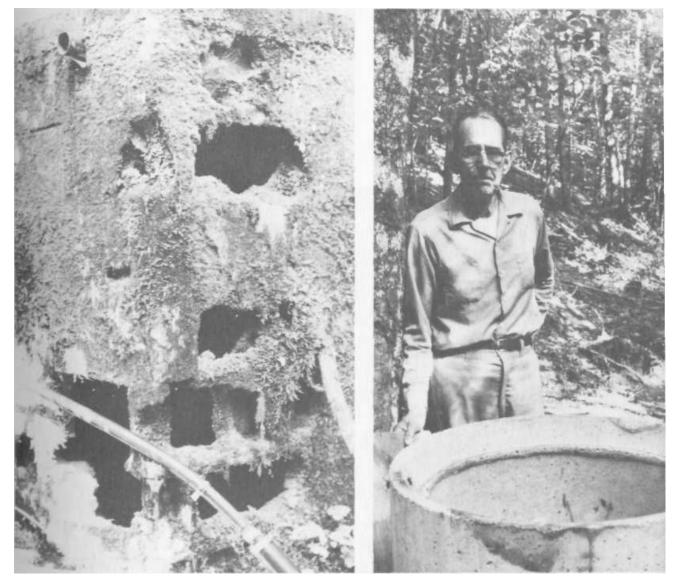
PLATE 301 Noel Moore's cementblock reservoir after a winter of freezing and thawing.
